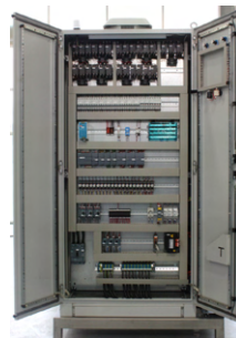
Electrical Panel, PLC, Sensor System (Temperature, Humidity, Pressure, etc. Safety Sensors), Electronic Equipment
